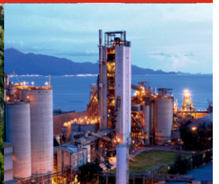
Oil & Gas Plant
